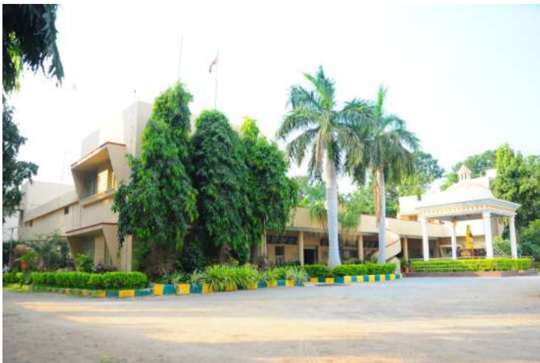
Head Office Main Building View
