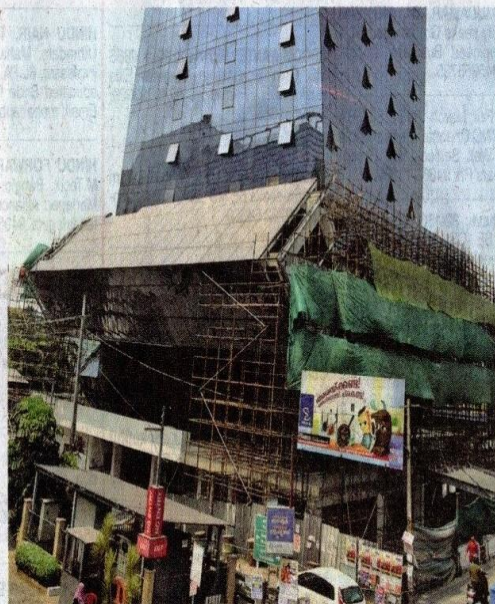
The International Cooperative Museum building is nearing its completion in Kozhikode.
